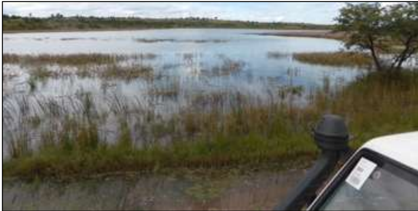
Dam – full at time of visit
