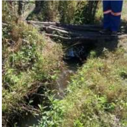
Water Channel (unlined)
