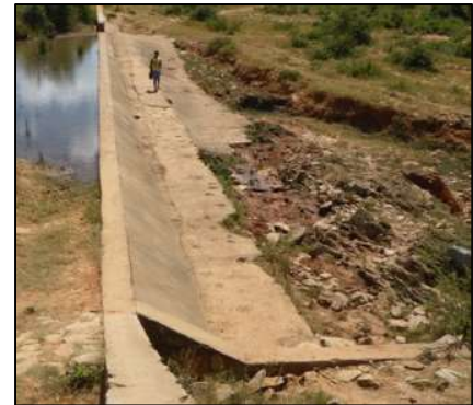
Spillway: manageable erosion
