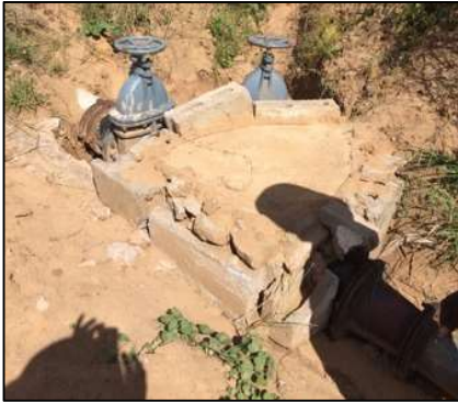
Piping works from pump station
