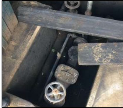
Piping works from pump station
