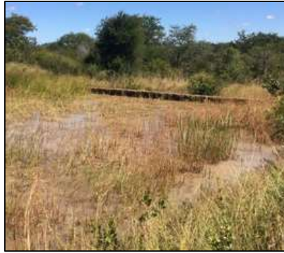
Spillway (silted)
