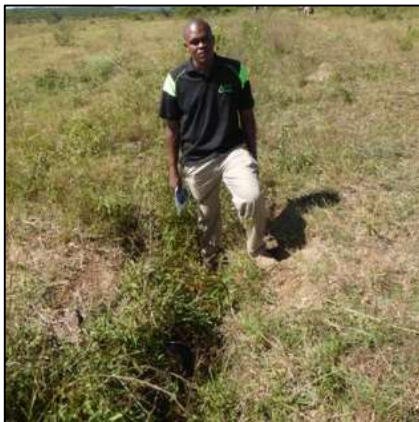
Main canal: overgrown but sound
